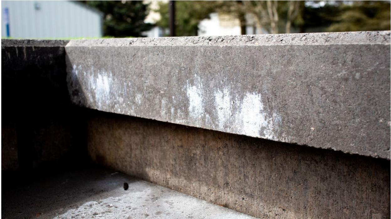
Likely, you're looking at efflorescence. Let me explain. When you boil it down, paving stones are just small blocks of concrete. The thing is, concrete doesn't dry quickly; it cures over time. During the curing process, calcium hydroxide (in the form of moisture) comes to the surface and combines with carbon dioxide in the air. Together, those two elements create calcium carbonate, which is also known as efflorescence.
