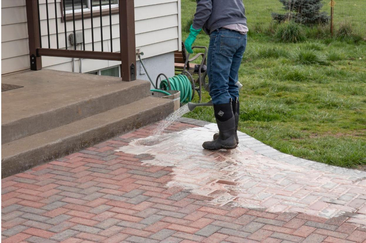
Muriatic Acid breaks down a micron thick layer of efflorescence on the surface of your paving stones, so it's common to experience some colored standing water or foaming on your pavers. Don't worry! It's normal. After rinsing, your hardscape will look as good as new.
