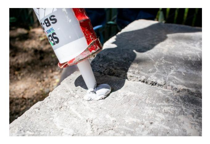
Apply the adhesive at least 2" away from the outside edge of the block to avoid glue from oozing onto the face of your column.
