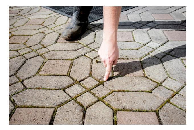
**First, scrape it with a flathead screwdriver.** We recommend that you place your screwdriver head in a vertical position so that while you break apart the moss, you don't scrape away the surface of your pavers.
