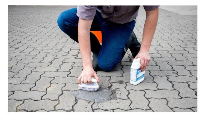
**Third, rinse using hot water.** While rinsing, we used our brush and scrubbed at the oil stain for good measure. Depending on the size and severity of your oil stain, you might consider using some additional elbow grease as well. If the stain is persistent, simply repeat the process another time or two and your pavers will be as good as new.
