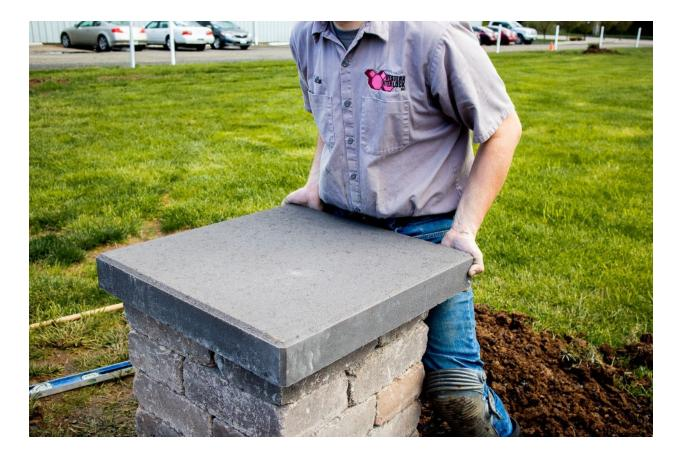
You'll want to measure all four sides of the cap between the wall blocks and the capstone edges to make sure your cap is perfectly centered. To do that, we just used our measuring tape and rubber mallet to make slight adjustments.
