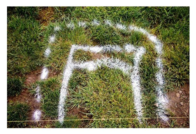
If you have columns that are going to be in line with one another you will want to set up a string line to use as a reference for level, straight, and square. Once your layout is marked, you can prepare the foundation. This all starts with digging.
