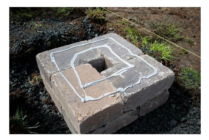
You will put beads or dots of glue on the top of every course while alternating or rotating the blocks to offset the seams. This is important for both aesthetics and structure.
