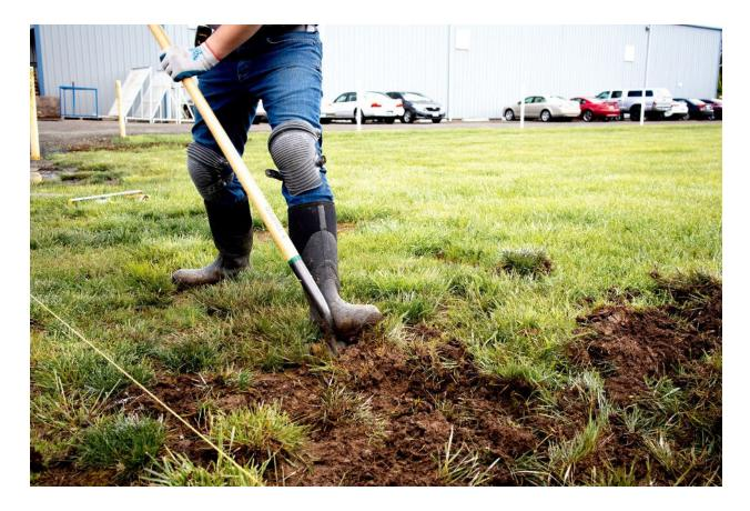
Dig out your outermost marked area about 8 to 10 inches deep. While the depth of your excavation is dependent on your desired overall height and the depth of your embedment, plan for at least 6 inches of compacted  $\frac{3}{4}$ " minus gravel and some breathing room.
