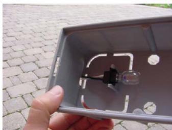
6. Run the low voltage cable which will supply power to the lights around the perimeter of your project. For installation with segmental pavers, you may set the cable atop the bedding sand under the border course of pavers to keep it from being damaged when digging in the yard and so it can be easily located. Remember to leave enough slack for connection of the light to the power cable.
