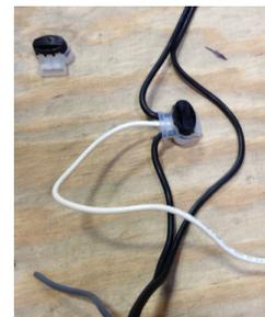
8. Examine the connectors and note there are three holes in each. The outside holes are for the power cable and the middle hole is for the lead from the fixture. Cut one side of the split power supply cable. There is no need to strip the insulation. Place each end of the cut power cable into the two outside holes in the connector. Push one of the cables from the light fixture into the middle hole. Visually make certain all three wires are pushed to the back of the connector.
