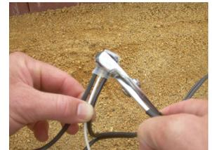
10. Repeat steps 8 & 9 with the other side of the power supply cable and the remaining lead from the fixture. You should end up with two connections per light as shown. **After all lights have been attached, plug in and switch on the transformer to test all connections.**
