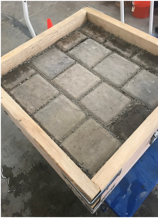
Photo #8 Step Bond as Installed
